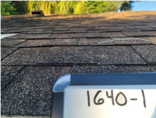
1640-1 Asphalt Shingle/Tar Typical Exterior Roof
